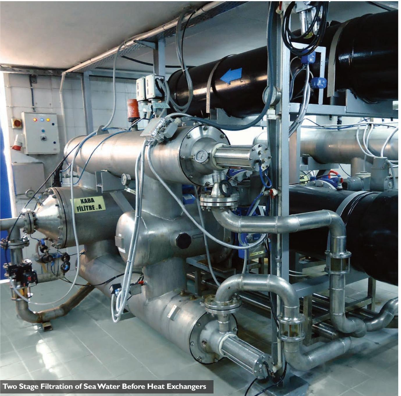
Two Stage Filtration of Sea Water Before Heat Exchangers
