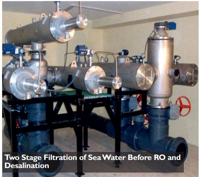
**Two Stage Filtration of Sea Water Before RO and Desalination**
